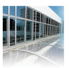
• The solar protection adhesive film SOL 251 allows overcoming the greenhouse phenomenon effectively. This film rejects 44% of solar energy and reduces the overheating keeping the external vision. It is a real factor for improved comfort.
